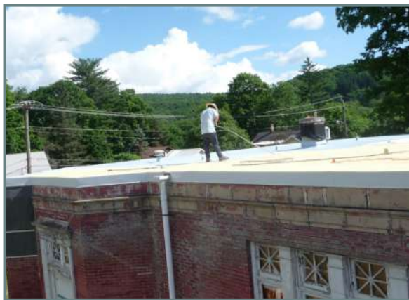
Sealing the Memorial roof.
